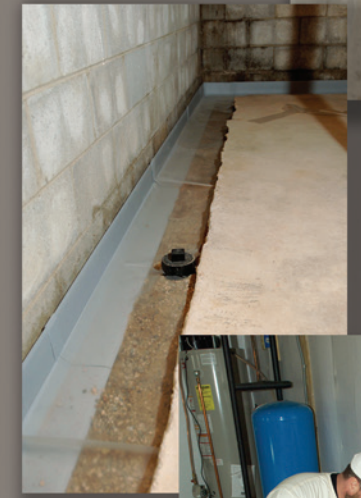
Photo shows optional 60 mil wall encapsulation product.
