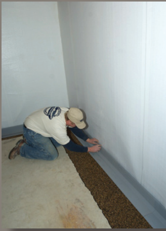
Photo shows optional 60 mil wall encapsulation product.
